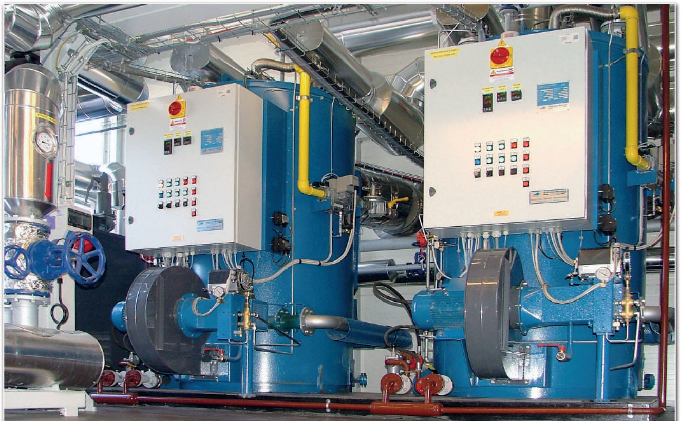
■ FROSTA Sp. z o.o. in Bydgoszcz - process boiler house, thermal oil
