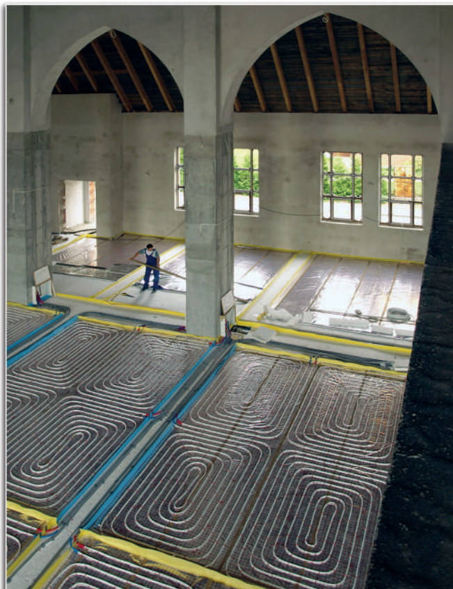
■ Floor heating under construction
