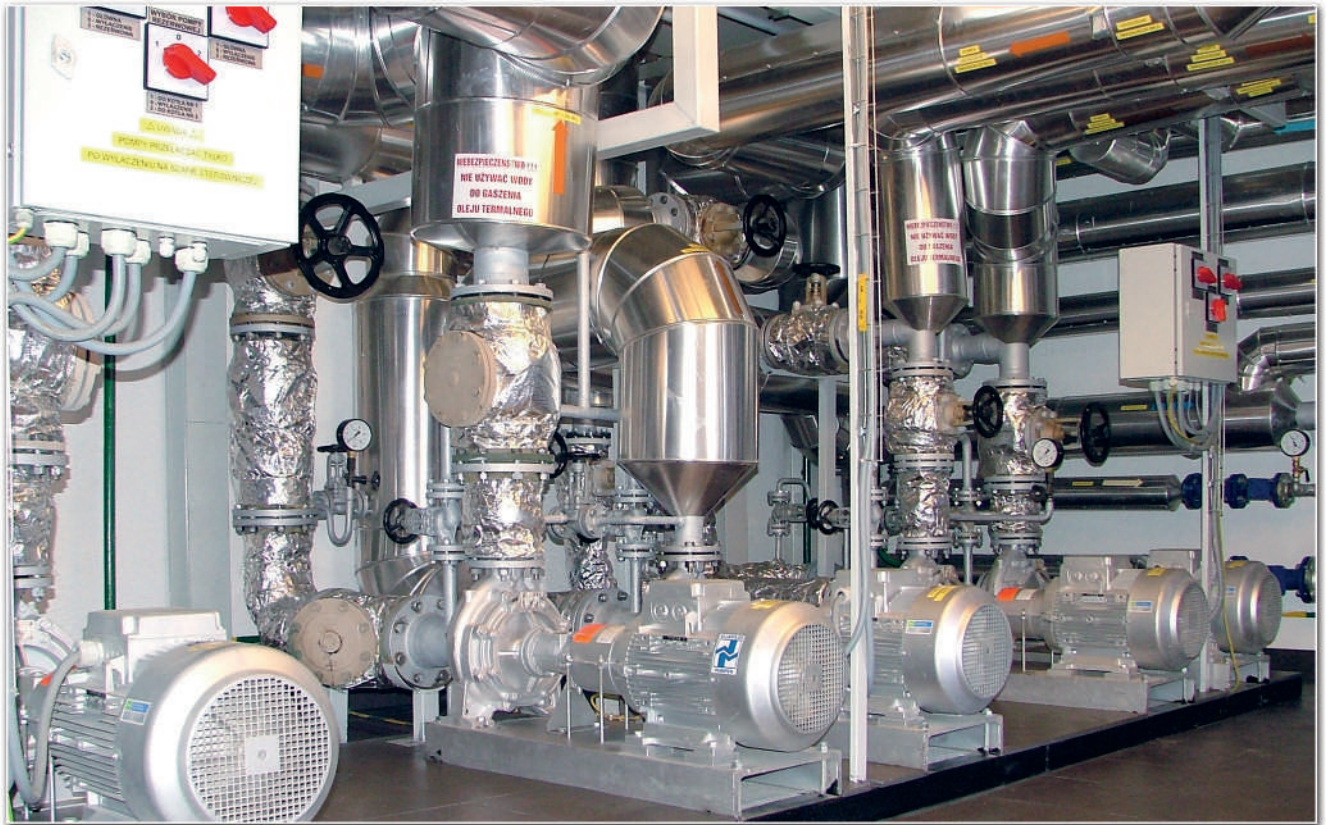
■ FROSTA Sp. z o.o. in Bydgoszcz - process boiler house, thermal oil
