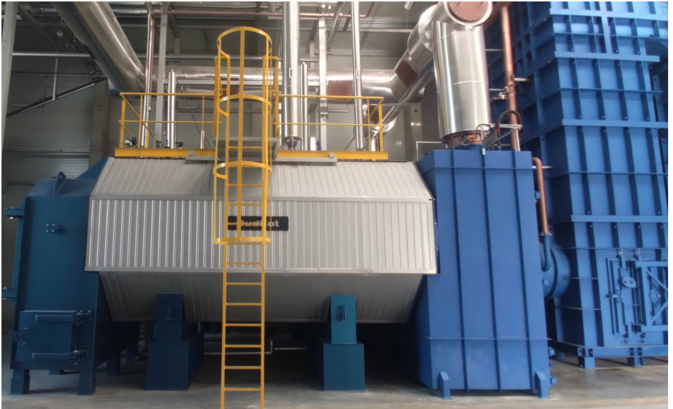
STEAM RECOVERY BOILER WITH Q = 1,5 \text{ MW}
