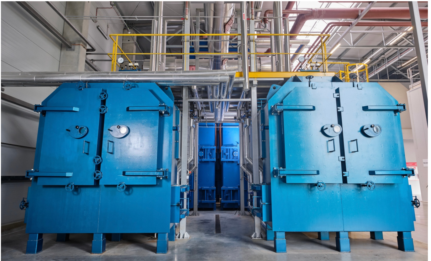
STEAM RECOVERY BOILER WITH Q = 3,0 \text{ MW}
